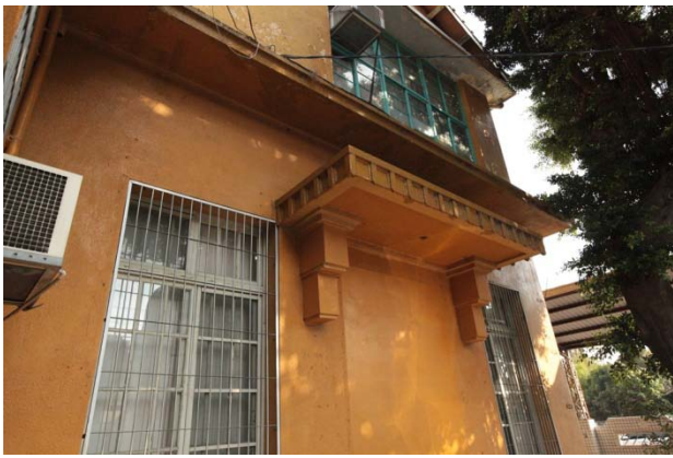
Fig 7 Photos of today's Wuri Municipal Government Building
