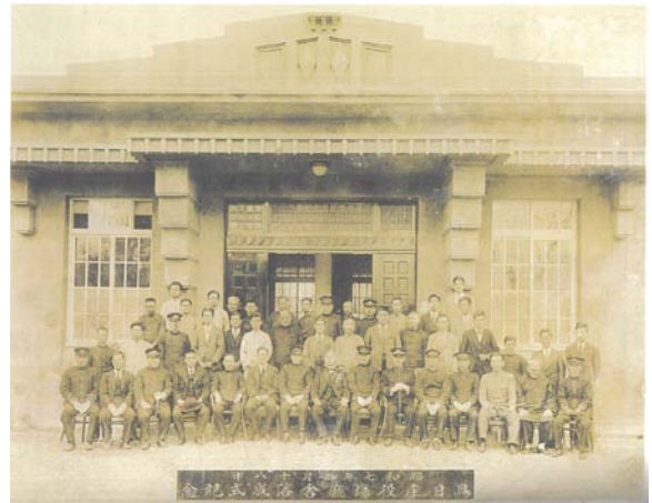
Fig. 1 Wuri Municipal Government Building in 1932
