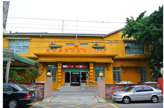
Fig.2 Wuri Municipal Government Building in 2014
