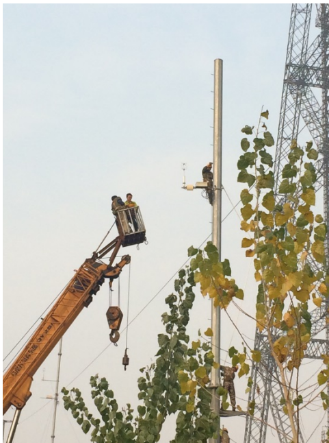
(a) Install wind speed meter
