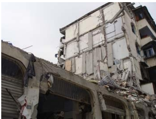
(b). Collapse of upper masonry layers.
