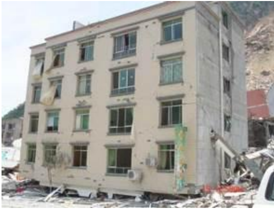
(a) Collapse of the bottom layer.
