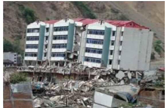
(b) Damage of the transition layer.
