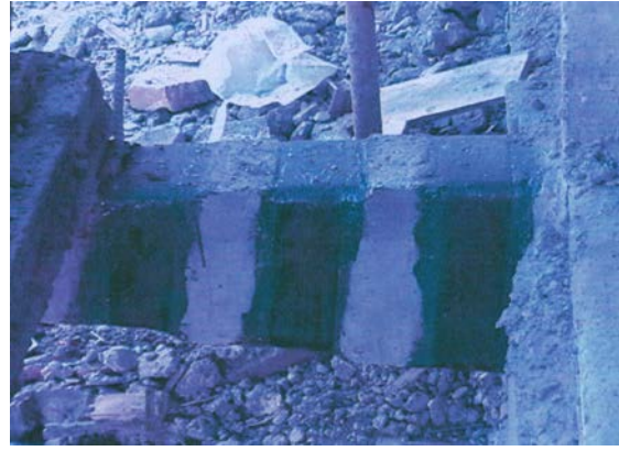
Fig.7 After Reinforcement Concrete Beam
