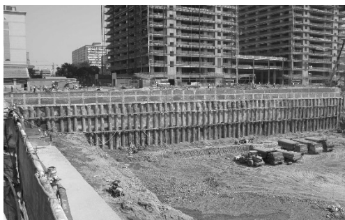
Fig.1 Row pile construction
