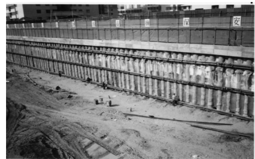
Fig.2 Row pile construction
