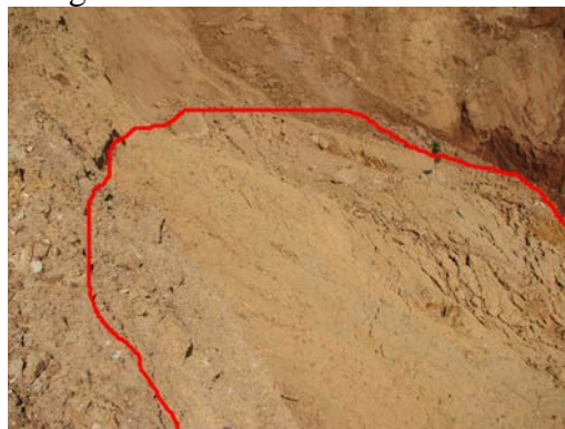
Fig.2 The loose landslide body in Ganshiya bauxite mine
