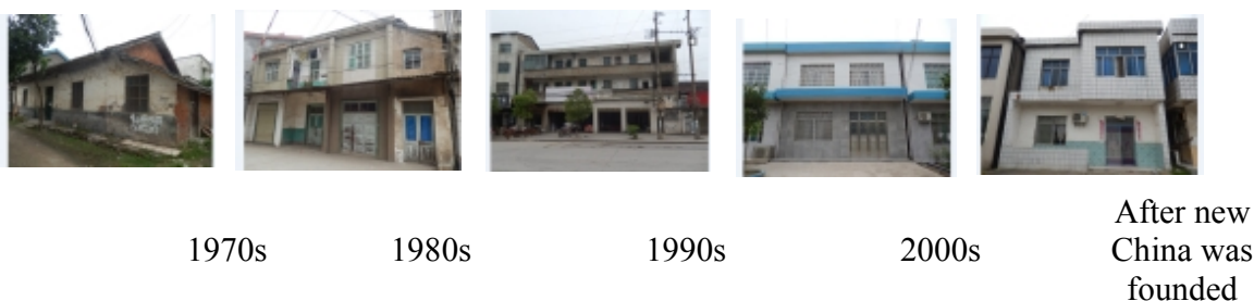
Fig. 15 Residential building during different periods
