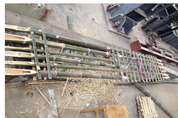
Fig.2 Binding bamboo reinforcement on the of site
