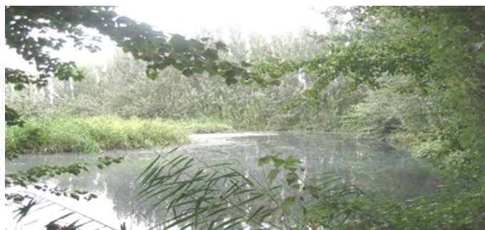
Figure 2. Constructed Wetland Sewage Treatment System in Pishan County
