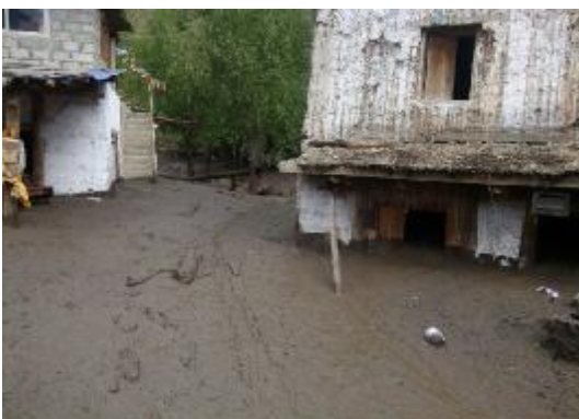
Fig.6 The debris flow destroyed houses
