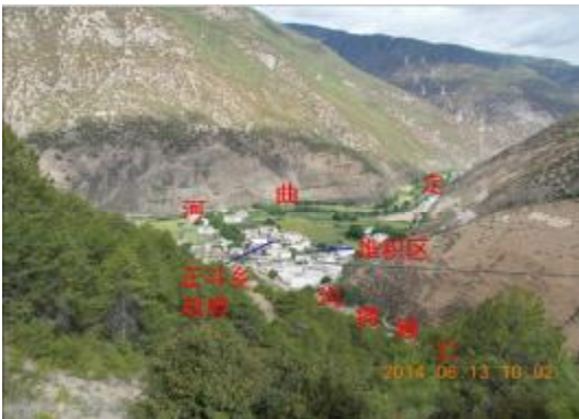
Fig.4 The danger zone of Reneyong gully
