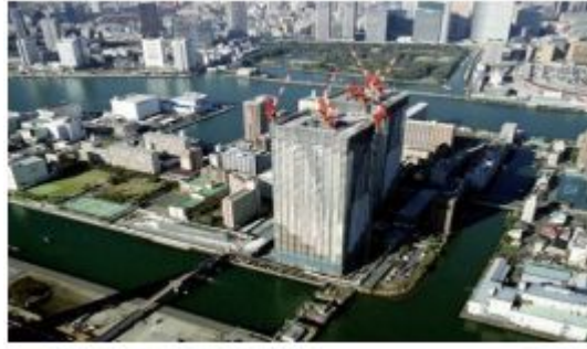
Figure 5 the world's tallest prefabricated concrete frame building
