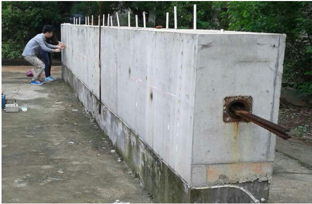
Fig. 3 The actual concrete member with corrugated pipe
