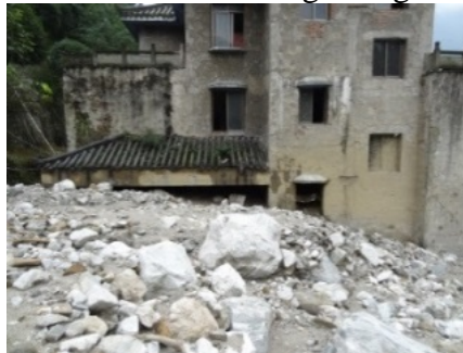
Fig.5 The buried house on the left bank of gully mouth
