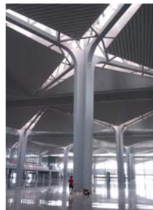
Fig. 6 Natural lighting of roof
