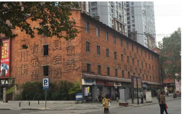
Figure 4. Status of existing buildings
