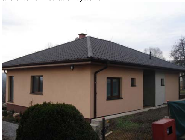
Figure 1. Measured timber house A.
