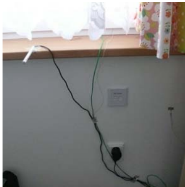
Figure 8. The location of the sensors in the construction.
