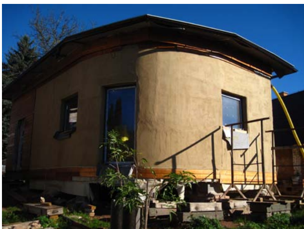
Figure 3. Measured timber house B.
