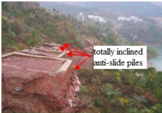
Fig. 6 Large deformation of slide piles on the Shijiapo Landslide in Badong County
