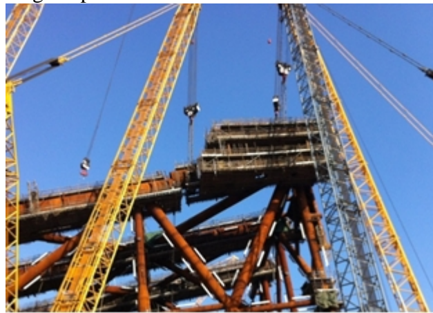
Fig. 9 skirt pile sleeve in position
