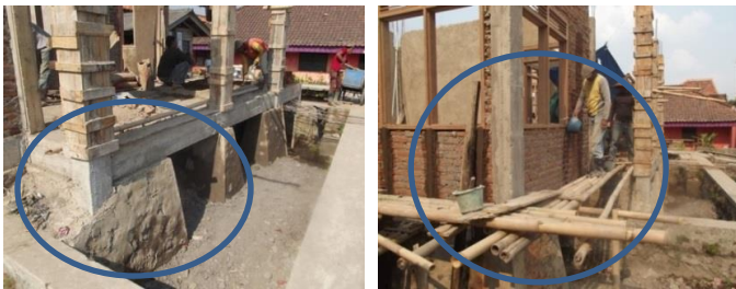
Figure 9. The stage house concept and optimizing natural lighting is adopted from traditional building of Kampung Naga Source: Research document, 2014
