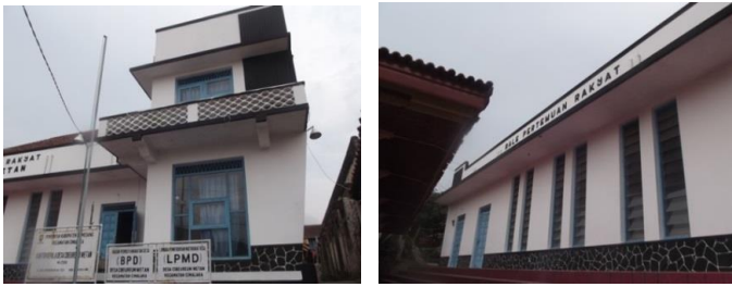
Figure 7 Community Center (Bale Desa) of Cibeureum Wetan, built by local worker in '70s Source: Research document, 2014
