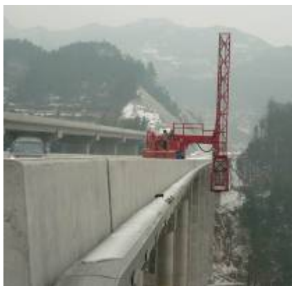
Figure 1 Bridge Inspection Vehicle
