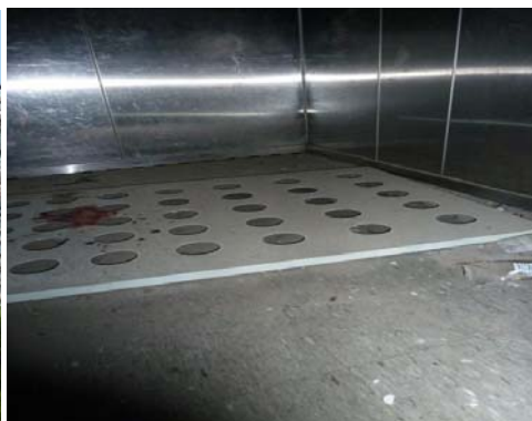
Fig. 2. Drop the car ceiling
