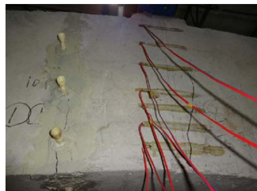
FIGURE V. THE GROUTING REINFORCEMENT CRACK DEVELOPMENT AFTER RELOAD
