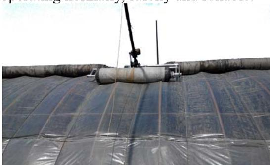
Figure 6 Seamless rolling machine rolling effect
