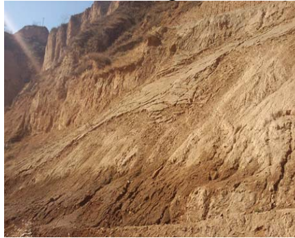
Figure 1 Landslide in sample point
