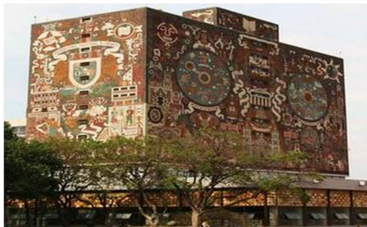
Figure.2 Mexico University Library Main Building exterior wall frescoes (Figure II)
