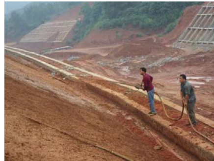
Fig. 2 Soil Spraying on the Experimental Slope
