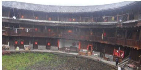
Figure 2 Wande Building, Meilin Village, Meilin Town
