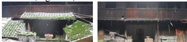
Figure15 Nanqing Building Figure16 The Jining Building
