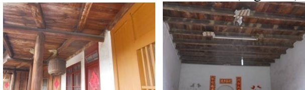
Figure 3 Huaxing Building, Jitou Village, Meilin Town
