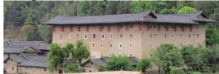
Figure24 Hegui Building, Pushan Village ,Meilin Town
