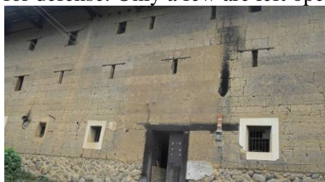
Figure 1 Huairen Building, Meilin Village, Meilin Town
