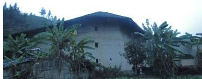
Figure27Nanxun Building, Shiqiao Village, Shuyang Town
