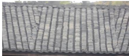
Figure 4 Scissor Tiling on the Rooftop of Round Buildings
