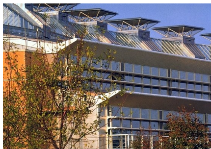
Fig.2 Air shaft on the roof
