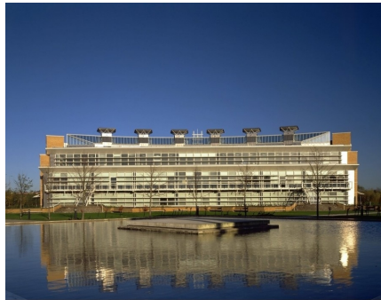
Fig. 1 Ionica Telecom headquarters
