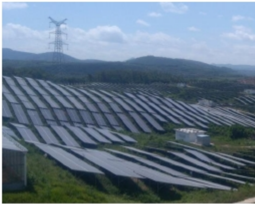
Figure 3. Photovoltaic panels and plant below
