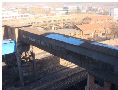
Fig.1 The external structure of 901 belt corridor
