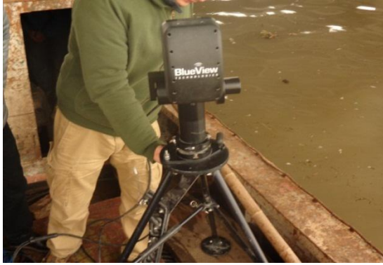
Fig.3 Sonar test on site
