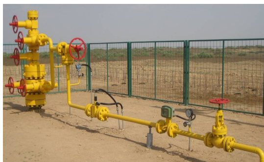
Fig.5 The well site in Sulige gas field
