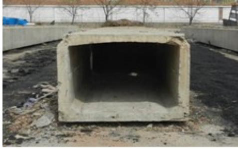
Fig. 2 The test void-box beam
