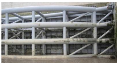
Fig.1 A sluice gate
