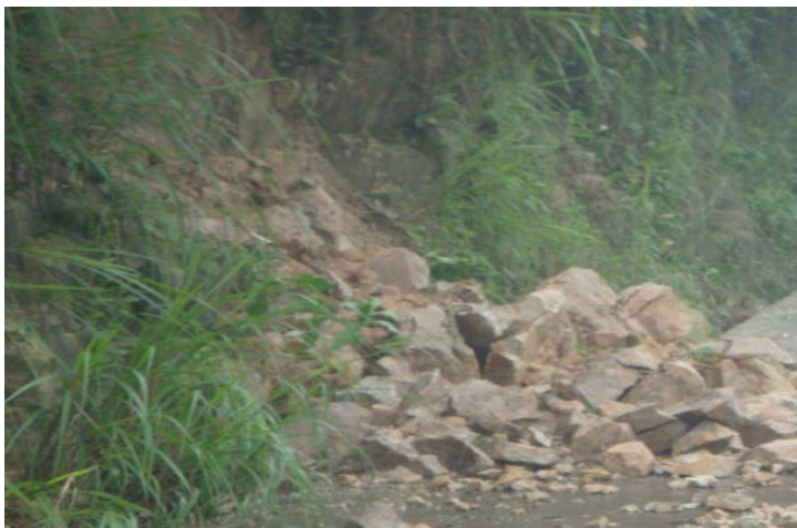
Figure 2.2 Highway Flood destruction Condition in Baiwukou Village
