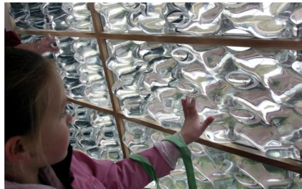
Figure 7. Water wall made of waste plastic bottles by University of Arizona in SDA2009
