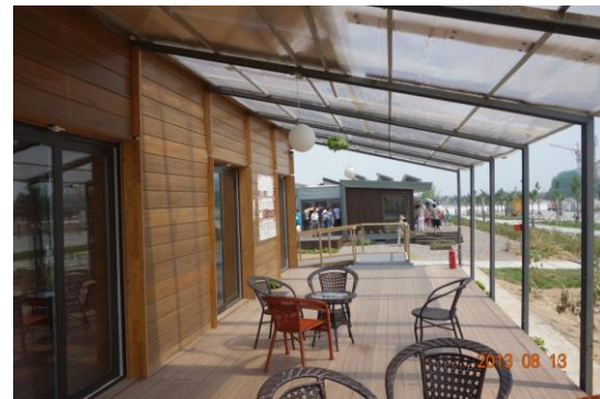
Figure 2. The south loggia in "Qi Ju"
