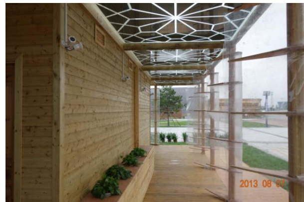
Figure 5. Ceiling ventilation in “River Sunvelop”
