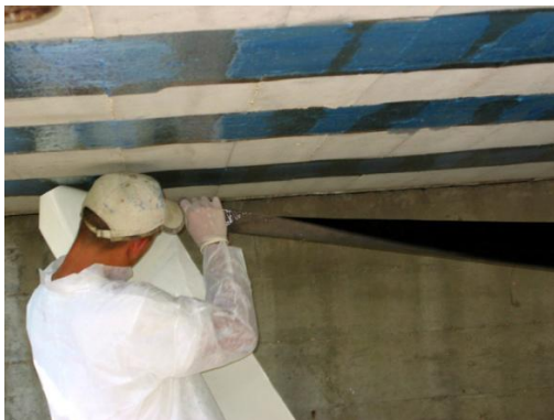
(c) Application of FRP laminates
