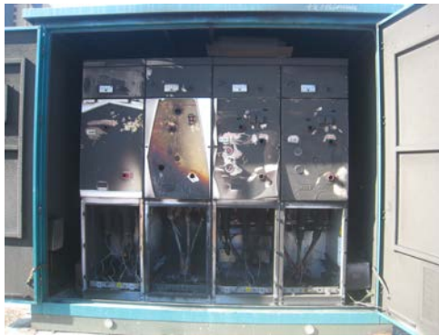
Fig.2 The pollution flashover of line ring main unit
