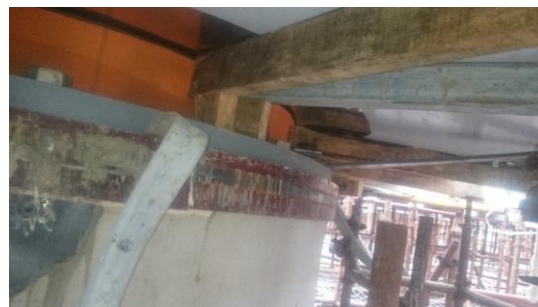
Fig. 14. The upper cover of the sliding isolation supported by the scaffold
