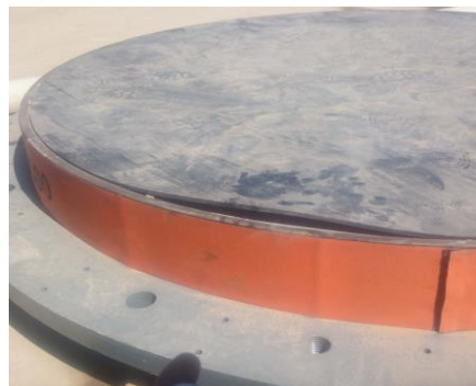
Fig. 6. The PTFE isolation bearing exposed to the sun is degummed and with bulge
