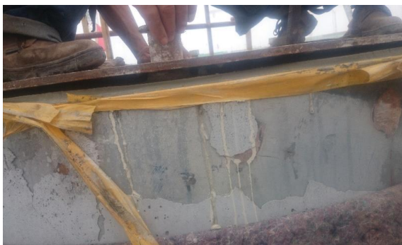
Fig. 5. The hollowing problem of the embedded board
