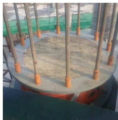
Fig. 10. The size of the felt is too small
