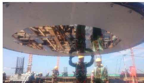
Fig. 12. Uncover the upper flange plate of the protective film during installation
