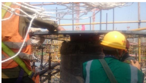
Fig.11. The placement of the sliding isolation bearing
