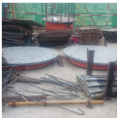
Fig. 9. The sliding isolated bearing is inverted
