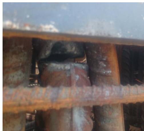
Fig. 4. The main reinforcement is cut
