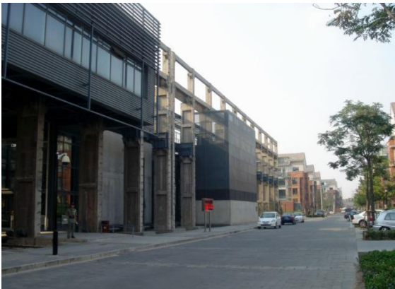
Fig. 2. The owner's club in residential area by reconstruction of old workshops
