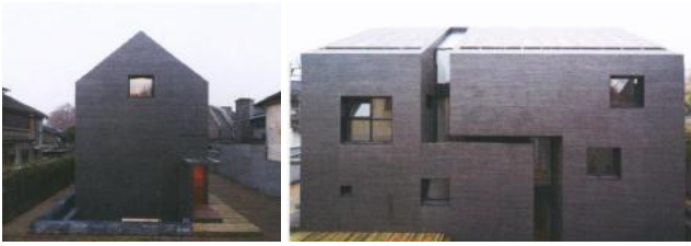
Fig. 7. Side Face and Right Face of House of Crack.
