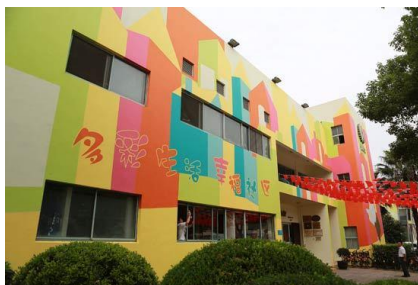
Fig. 2. External wall of Vanke service center
