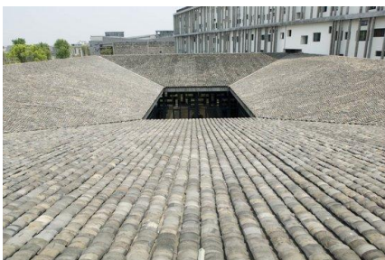
Fig. 2. Courtyard space on Xiangshan campus.
