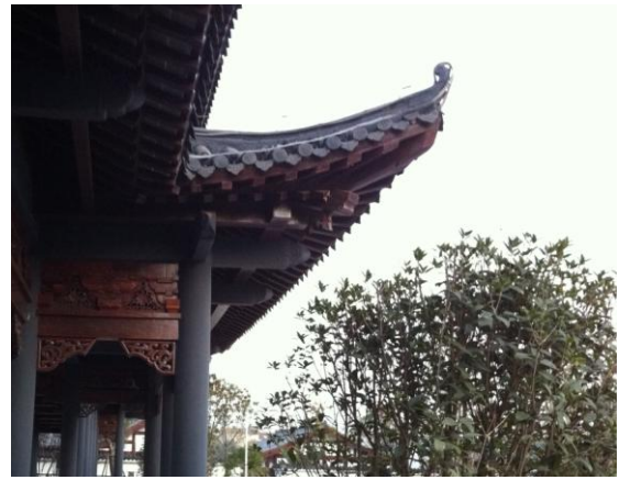
Fig. 2. Cornice in Chinese ancient architecture
