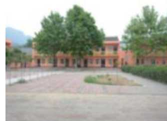
Fig. 8. Interior of Hepo Village Nursing Home.
