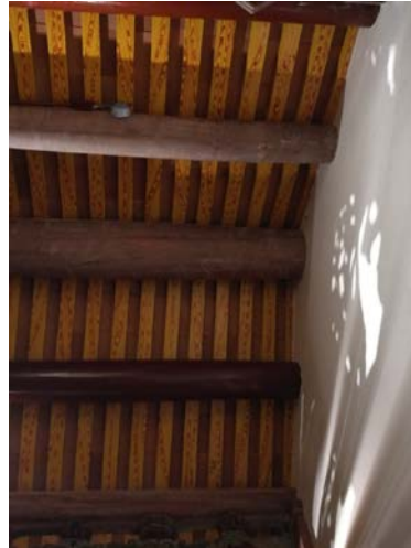
Fig. 1: Purlin used for replacement after restoration of Jiang's family temple
