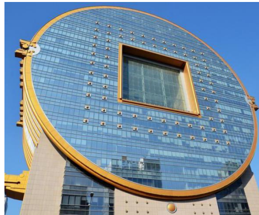
Fig. 2. Fangyuan Building (The figure is from network).
