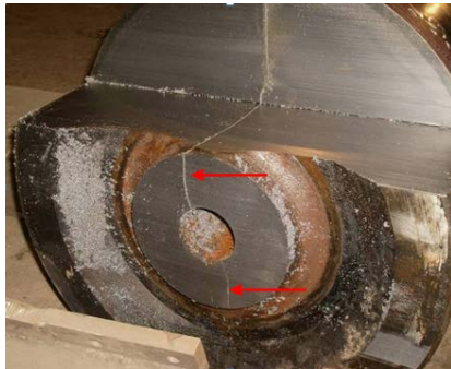
Fig.4. The crack passes through the roller section
