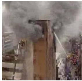
Figure 3a Smoke out of the ventilation Windows on the top floor
