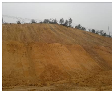
Fig. 1 Situation of test slope before construction
