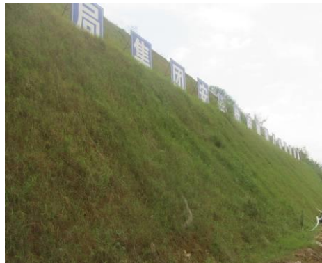
Fig. 8 Whole greening effect of comparison slope (22 months after construction)
