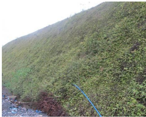
Fig. 7 Whole greening effect of test slope (22 months after construction)
