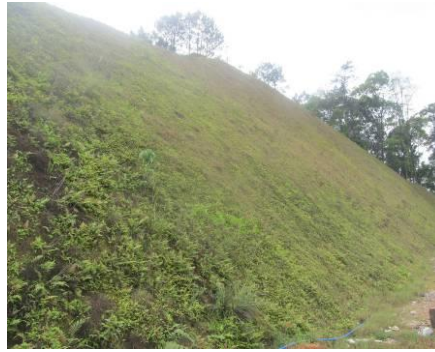
Fig. 2 Whole greening effect of test slope (22 months after construction)
